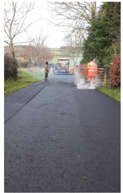
Road refurbishment at Tobberpatrick Aughrim - Storm Damage Funding
